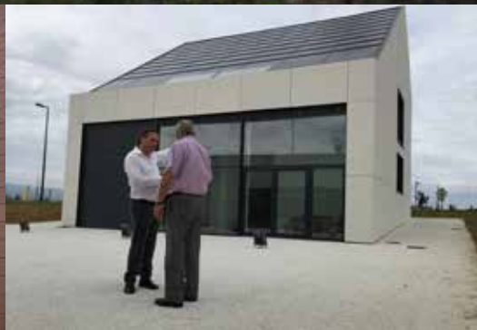
Smart House - R&D Centre - Venette, France
