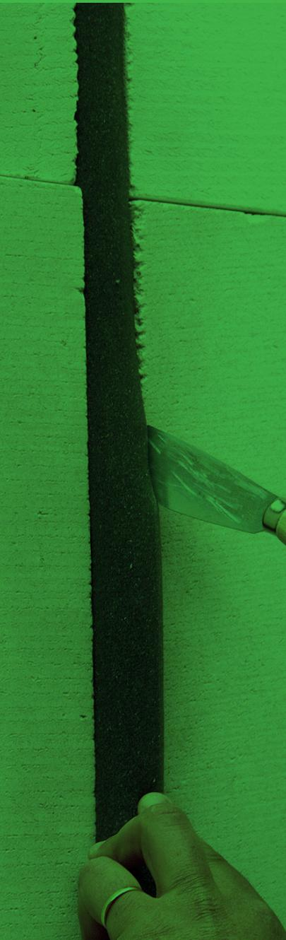
To apply the sealant with the correct depth, a backer rod is used (see drawing)
